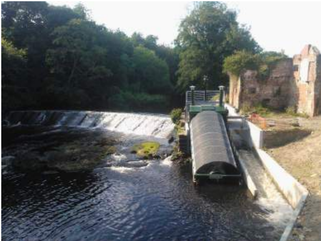
Figure 2: Floodproof screw installed at Goldsborough, North Yorkshire
